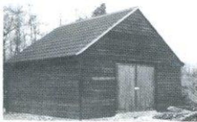
The new club storehouse situated at Bell Wood Fishery
