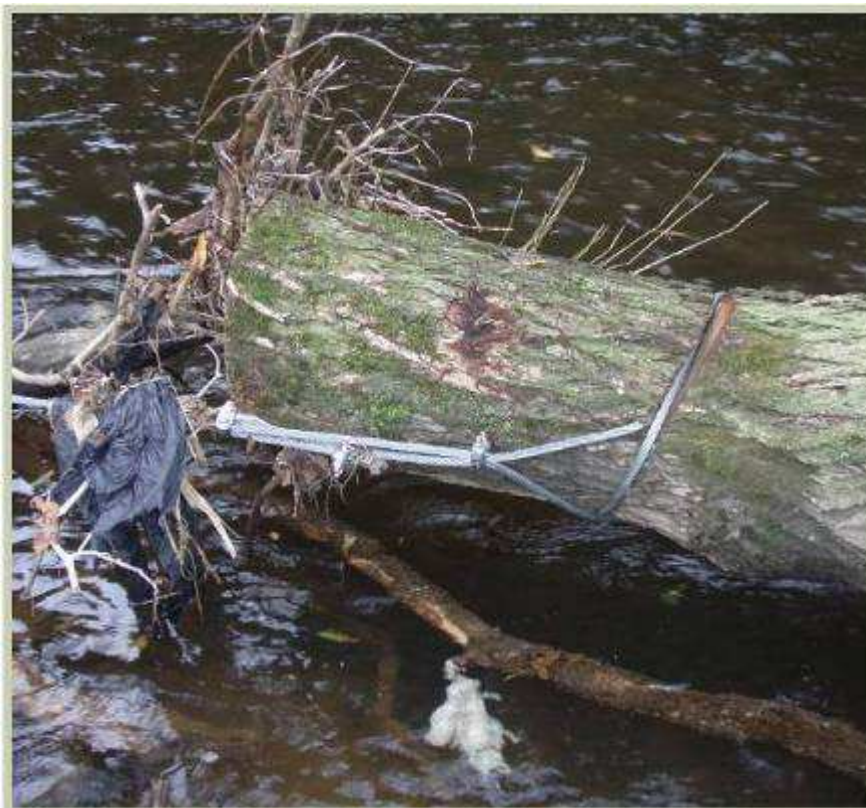
Figure 13. Cabling for a tree kicker.
