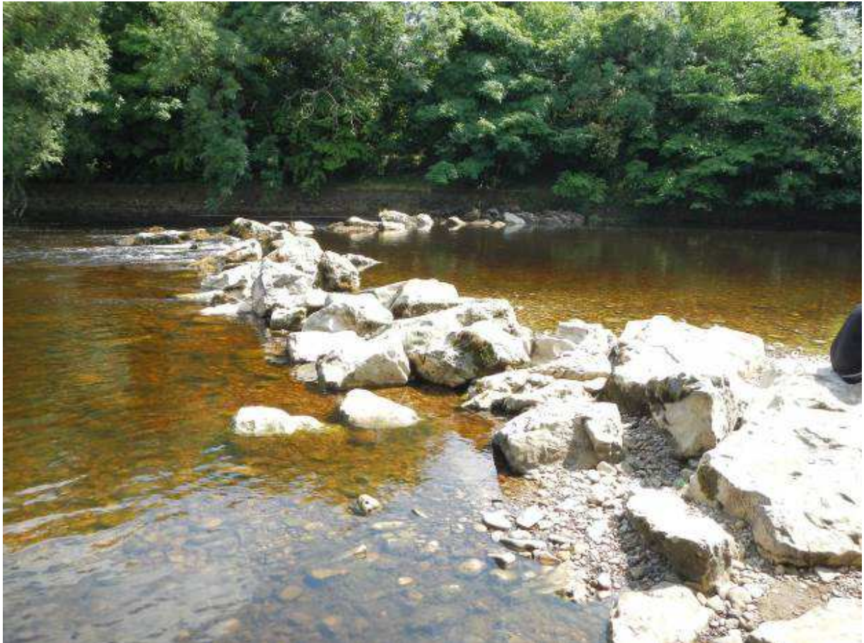
Figure 6. Downstream facing weir. Ideally this structure would have been created facing upstream and had a notch in the middle to allow bed material to pass through the section and create beneficial scouring.
